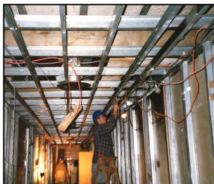
An engineer repairing the fire damaged corridors
